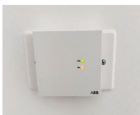
Figure 17. Air temperature, relative humidity, and CO 2 concentration sensor located in the living room to monitor the air quality.
