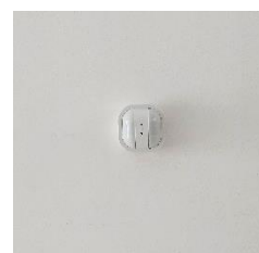
Figure 18. Room presence and luminance sensor integrated on the ceiling of the living room.
